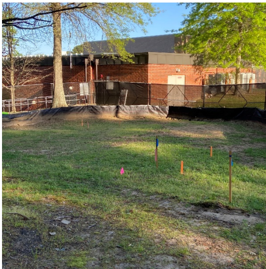
Power Locates and Building Layout
